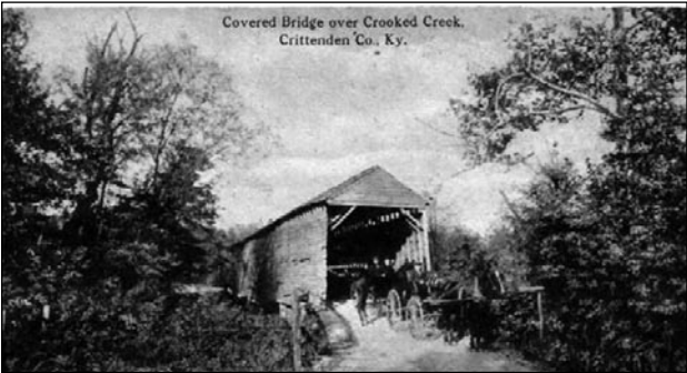
This postcard preserves the history of the Crooked Creek bridge. It shows Mr. and Mrs. Fred Gilberts crossing the bridge in its early days before the weather took its toll on the structure.
